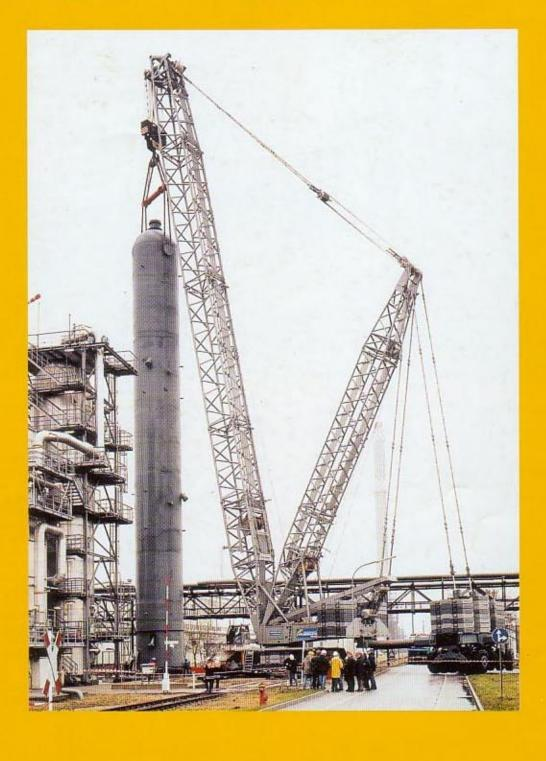
A heavy-duty lift out of the ordinary was performed at a refinery in Schwedt on the river Oder, close to the Polish border. A team of the Austrian Felbermayr group proceeded with the Liebherr heavy-duty crawler crane LR 1600/1 to the site in order to position a
